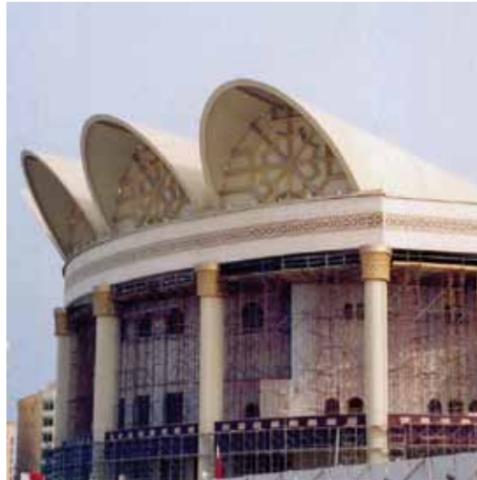
Architectural roof structure BFG International Ltd. Bahrain Firepel® K133
